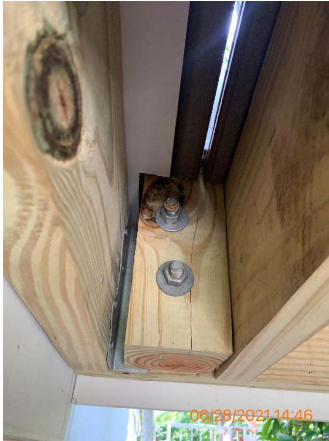
Figure 19 - All Guard Post connections need to be constructed per FFC Detail_Guard Post Connections Pages 20 21 and 24 Figures 37 38 and 40
