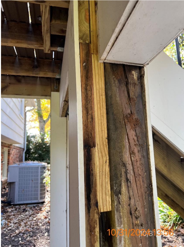
Figure 13 - Another snapshot of altered existing post
