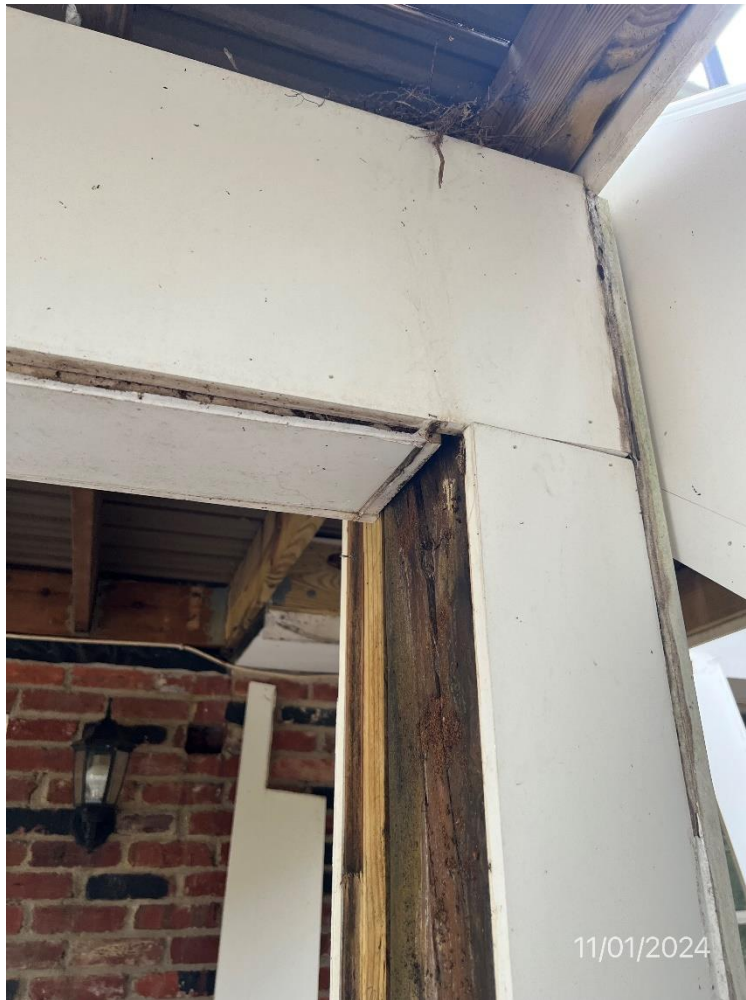
Figure 17 - Another view of the post closest to the patio with support beam to its left that is open on the top where debris and water are collecting and effecting the top post's cracking and deterioration
