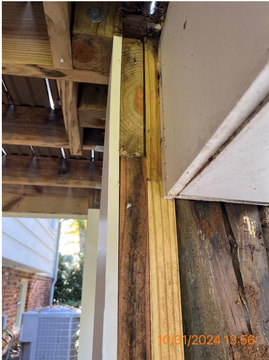
Figure 14 - Original post with alterations with rot and cracking under white PVC support beam that runs across the front of deck
