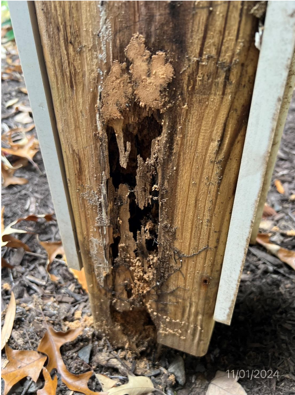
Figure 10 - Another close-up of rotting post
