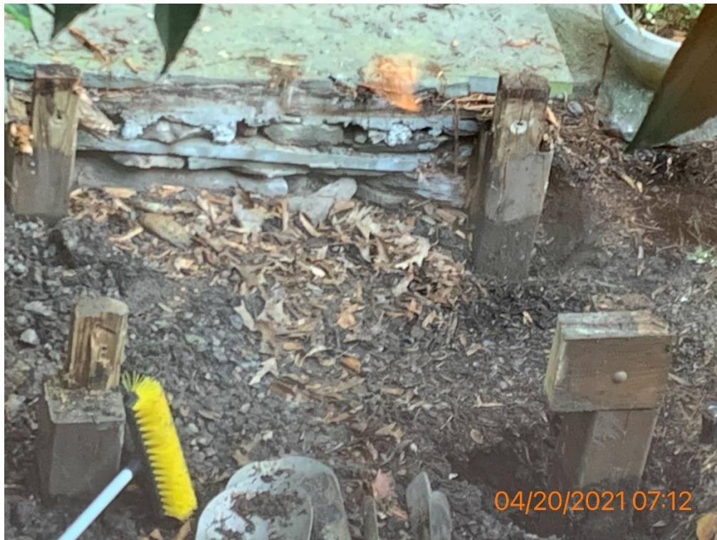
Figure 3- Demo photo of original deck posts
