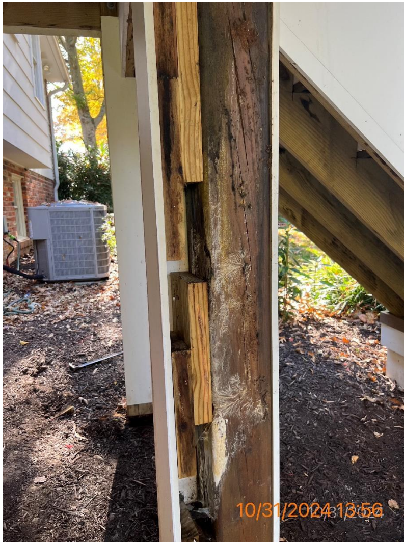
Figure 16 - Close up of top section closest to patio post to beam connection not correctly installed per violation FFC listing
