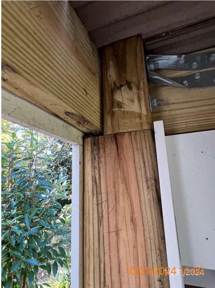
Figure 12 - Close-up of the top section of the support post that is rotted under deck - Guard Post Connections and Post to Beam connection violation
