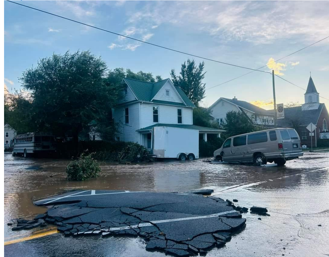
Pictured: Flood Damage to Single Family Home and Road in Washington County; courtesy of VDEM
