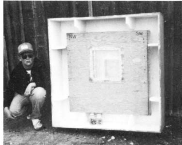
Fig. F.3. The Top and Four Walls of the Multi-Purpose Emergency Exit Housing, Nested Together to Save Storage Space.
