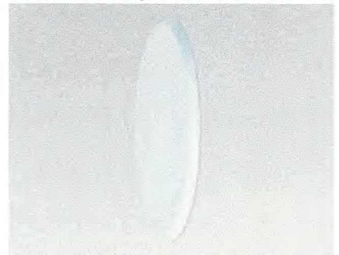
Concealed Sidewall Sprinkler
